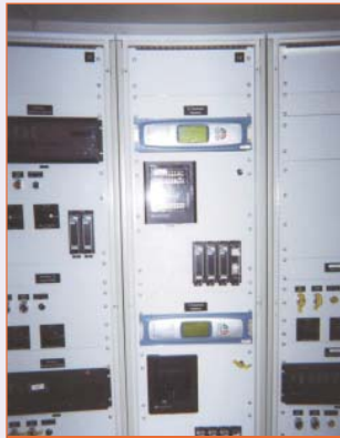
DRMCC site installation
